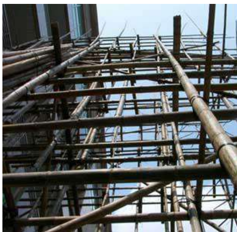
Fig- Bamboo scaffolding
